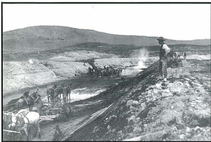
Teams of horses pull "Fresno plows" to excavate the division two of the main canal for the Klamath Project on February 13, 1907. Hot springs in the bed of the canal send up clouds of smoke in the cold winter air.
