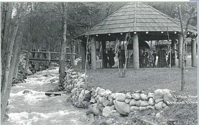
The creekside rock walls demonstrate an early attempt to separate the flood-prone creek from the landscaped portion of the park.
