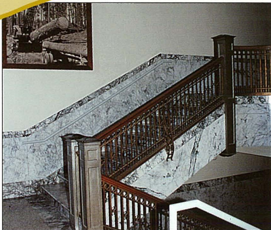
Up-to-date iron stair railings were provided by the Woodbridge Ornamental Iron Co. of Chicago. The railings were fitted between stainless steel newel posts. The inside stairs, wainscoting and corridor door casings were all made of Alaska marble, brought down from a Kodiak quarry.
