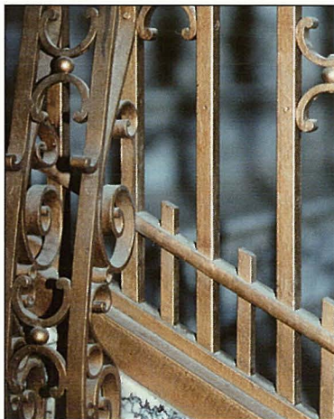
Up-to-date iron stair railings were provided by the Woodbridge Ornamental Iron Co. of Chicago. The railings were fitted between stainless steel newel posts. The inside stairs, wainscoting and corridor door casings were all made of Alaska marble, brought down from a Kodiak quarry.
